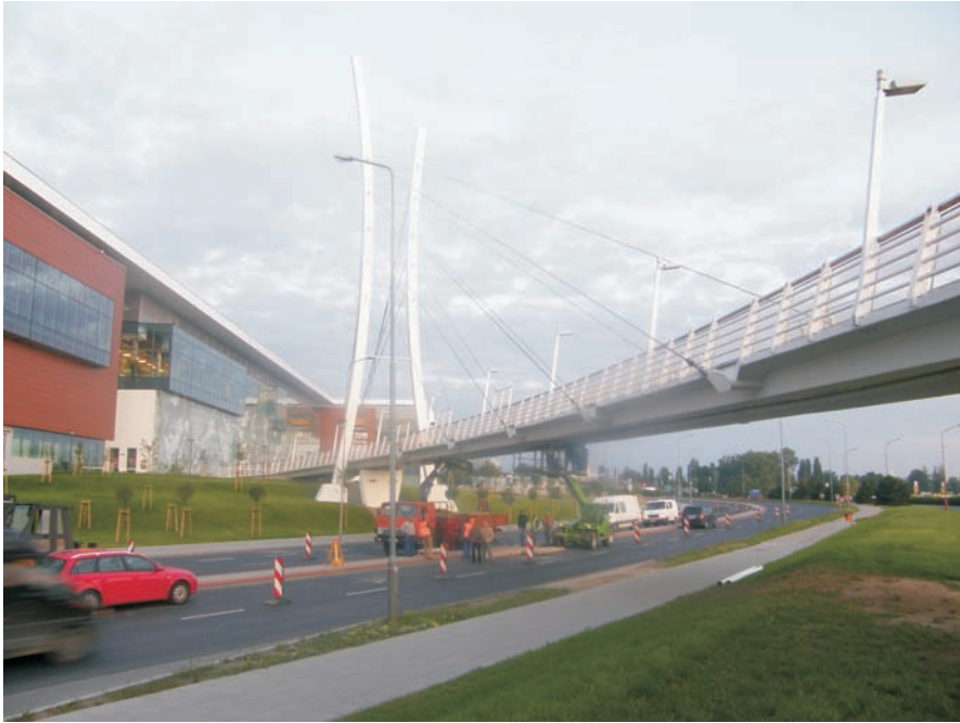
Fig. 8. View of the footbridge at the Malta Shopping Center in Poznań.
