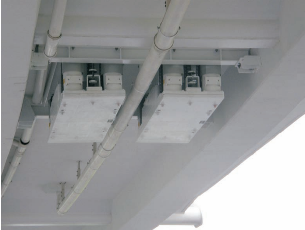
Fig. 10. TMD from GERB at Malta center in Poznań.
